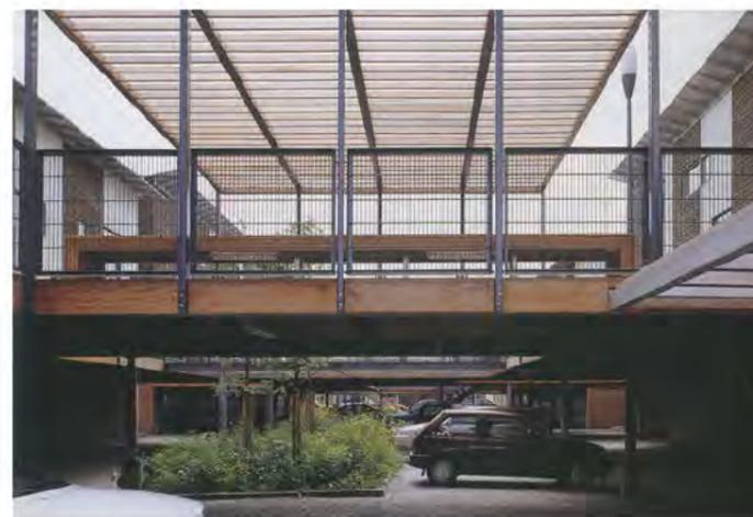
Fig. E12. Example of undercroft parking below a raised amenity deck.
