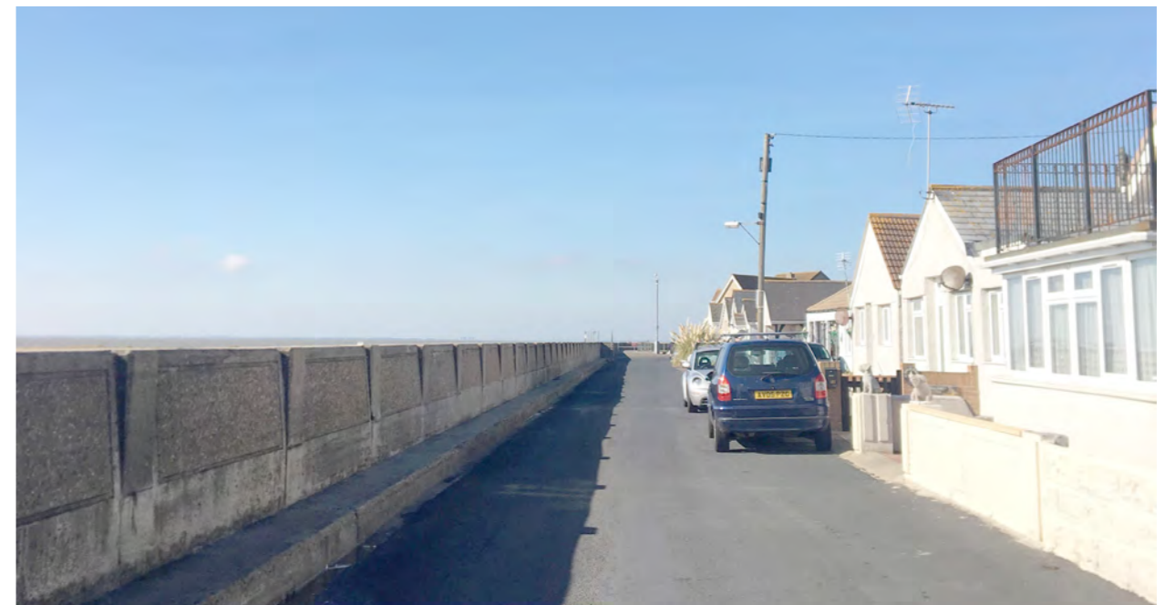
Fig. C33. View of Village seafront (DU3) - current condition
