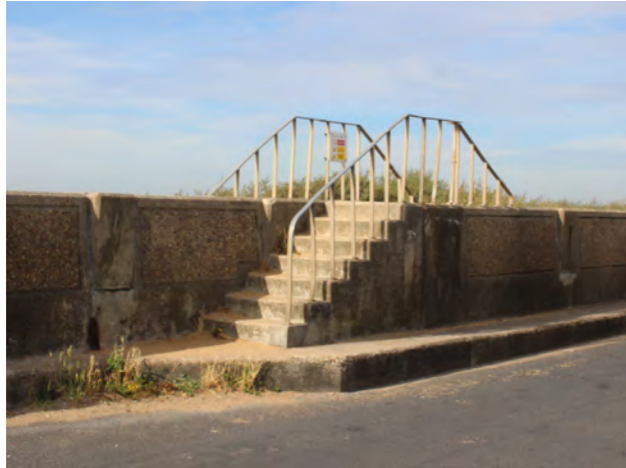
Brooklands seafront - sea wall varies between approx. 1.5-1.9m above the road level.
