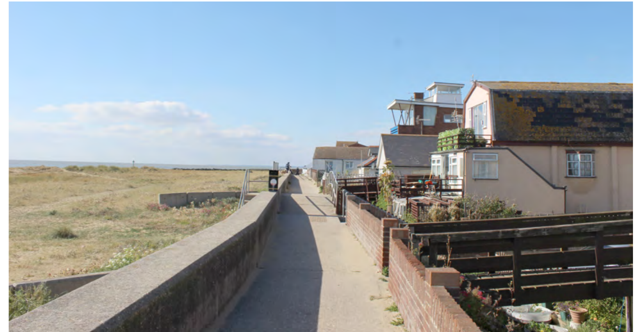
Fig. C18. View of Village seafront (DU3) - current condition
