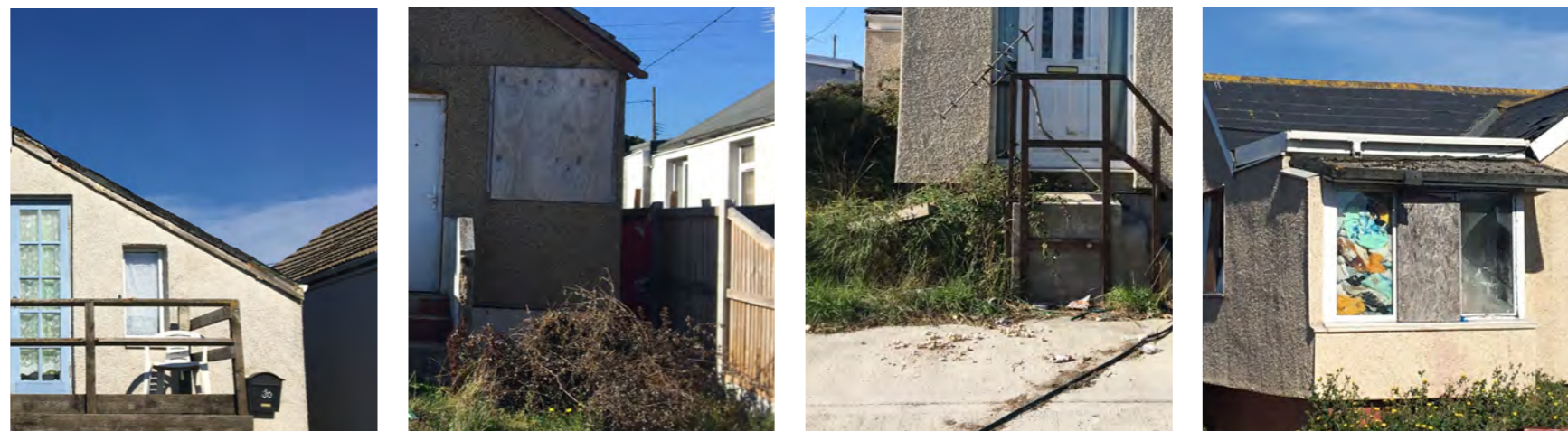
Fig. 49. Examples of occupied housing in poor condition.
