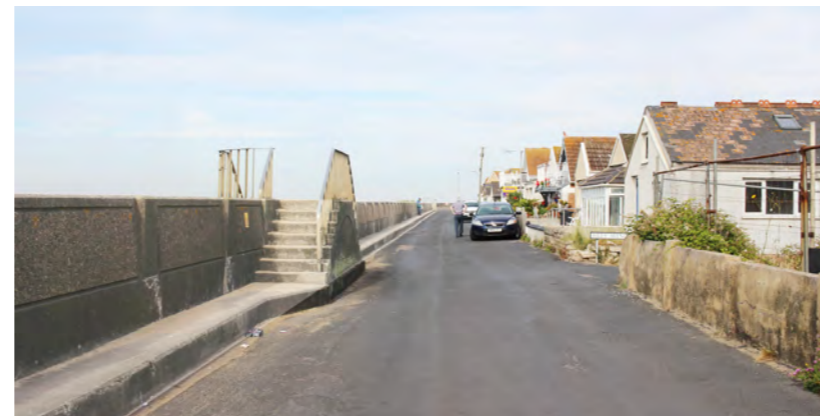
Fig. 75. Photograph of current condition of Brooklands
