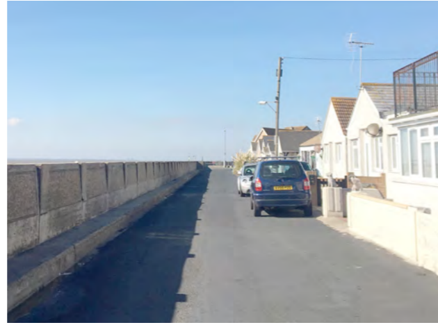
Brooklands seafront - sea wall varies between approx. 1.5-1.9m above the road level.
