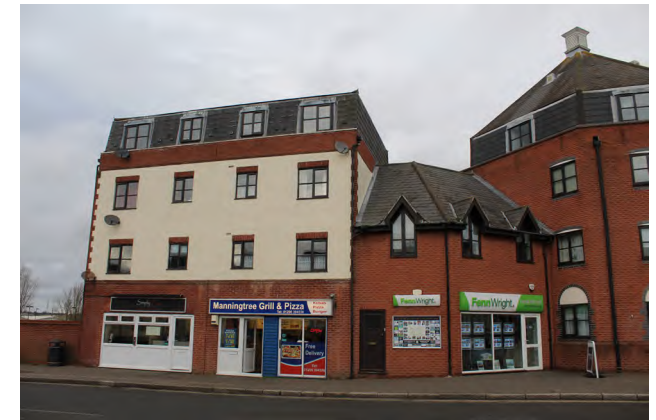
Figure 58 Blue brick window heads and sills
