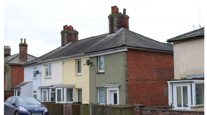
Figure 128 Examples of natural slate roofs within this Character Area
