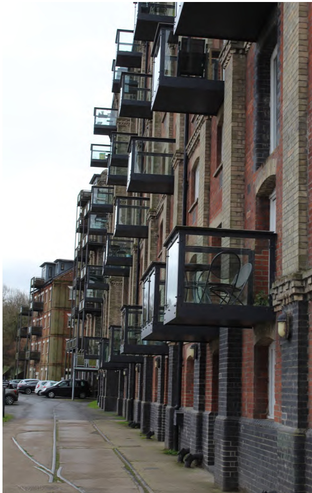
Figure 114 Rear of Maltings and Kiln 1 overlooking the River Stour with recent balcony editions. The trackways have been retained.
