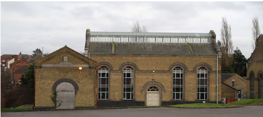
Figure 70 Pump House, Lawford Water Works
