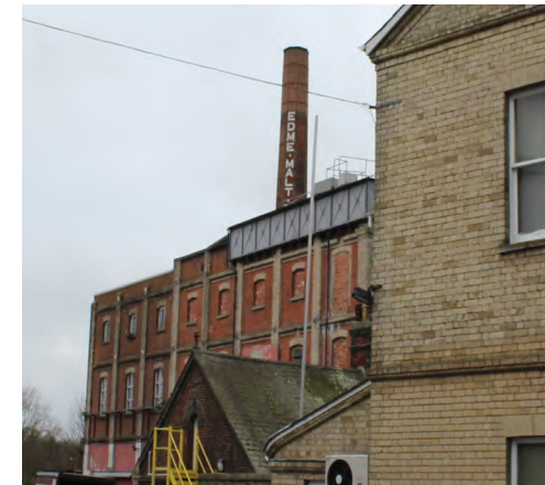
Figure 26 Rear of EDME Malt Extract Factory and Chimney, High Street
