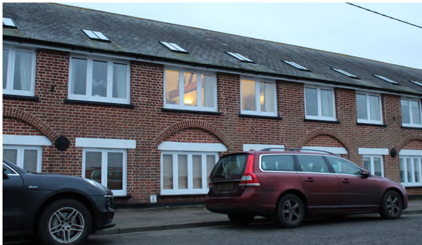
Figure 76 1-10 Brooks Malting with partially infilled arches
