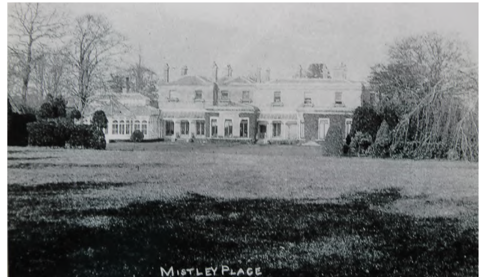
Figure 10 Photograph of Mistley Place. Building demolished after WWI. (JBArchive)
