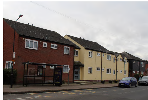
Figure 57 Same modern development of Bendalls Court fronting Station Road
