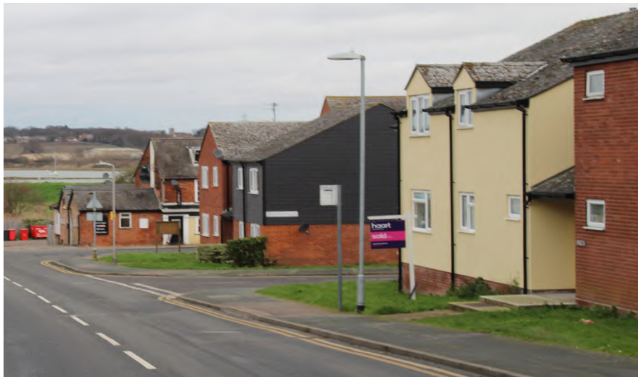
Figure 53 Flats along Colchester Road and entrance to Bendalls Court, The Skinners pub in background
