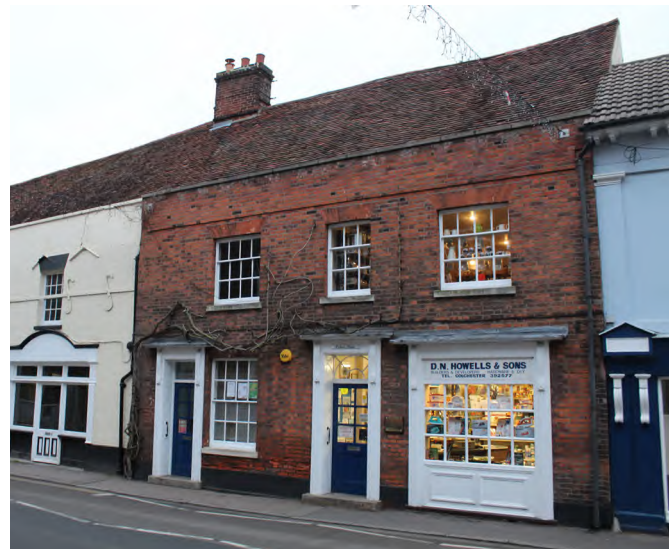
Figure 148 Historic shop frontage, Manningtree
