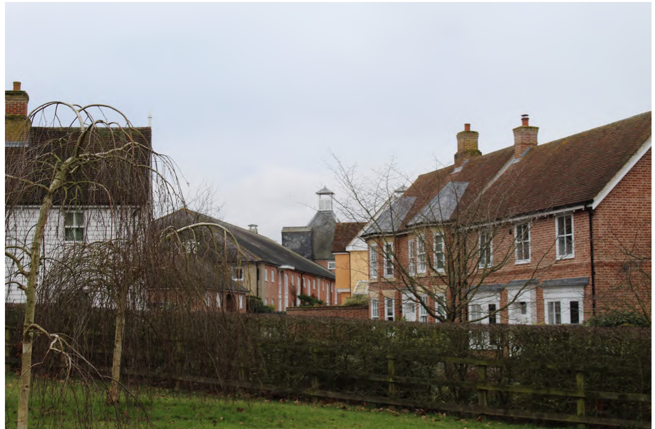
Figure 74 Listed maltings buildings at centre of development
