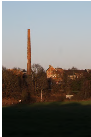
Figure 120 EDME Chimney from Green Lane
