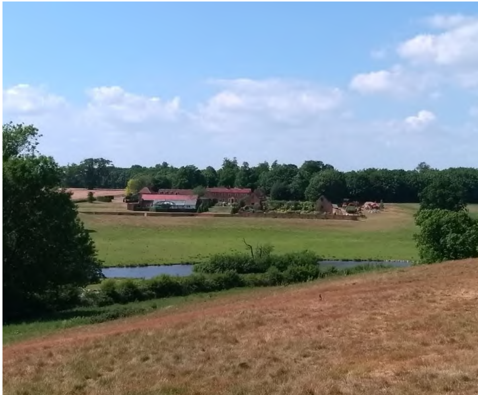
Figure 83 Grade II listed buildings at Dairy House complex including stables, dairy, brewhouse and cowhouse
