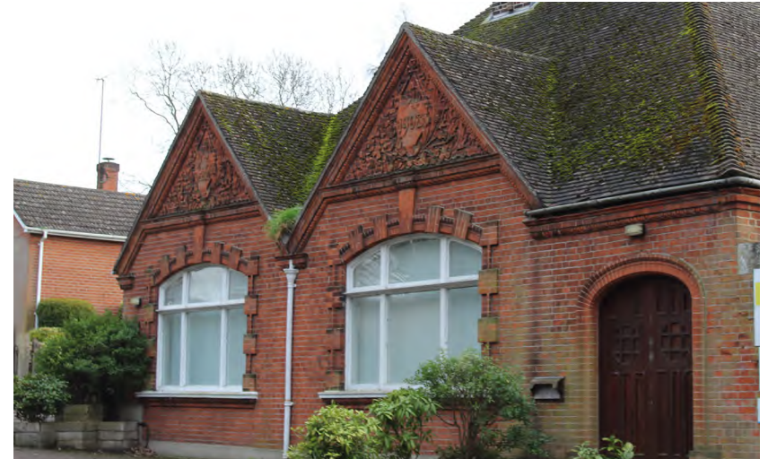
Figure 71 The Bungalow, Lawford Water Works
