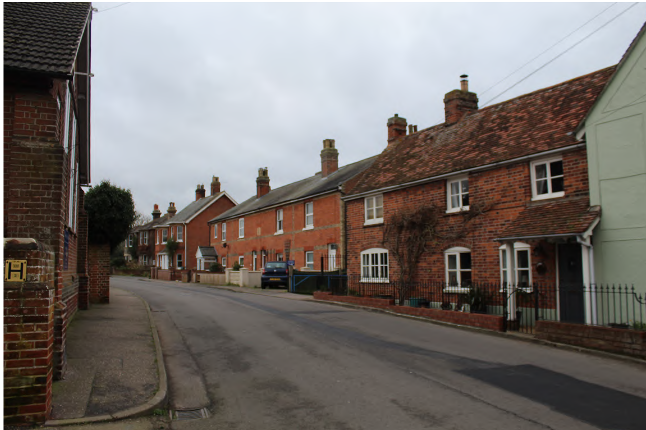
Figure 62 View south along Trinity Road
