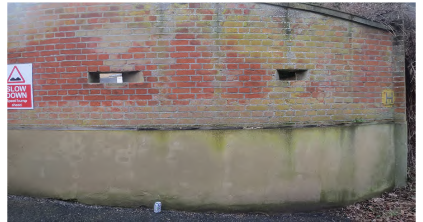
Figure 72 Boundary wall with loop holes, Lawford Water Works
