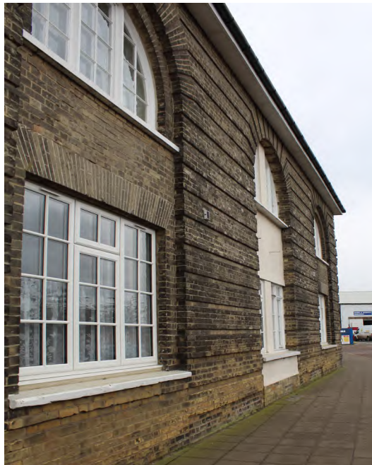
Figure 33 Grade II listed former warehouse to the east of south street
