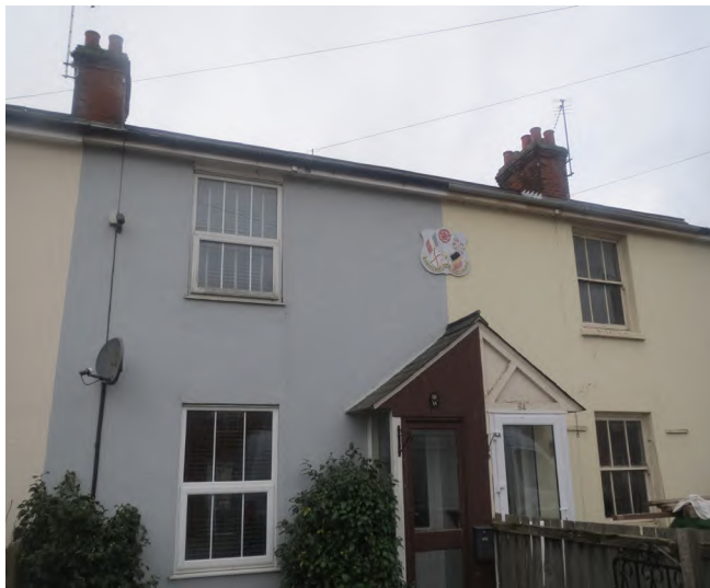
Figure 150 Visual comparison of historic retention of sash windows (right) and modern replacements (left)
