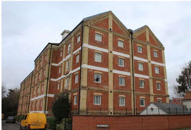
Figure 124 Grade II listed maltings, Nos. 3 and 4
