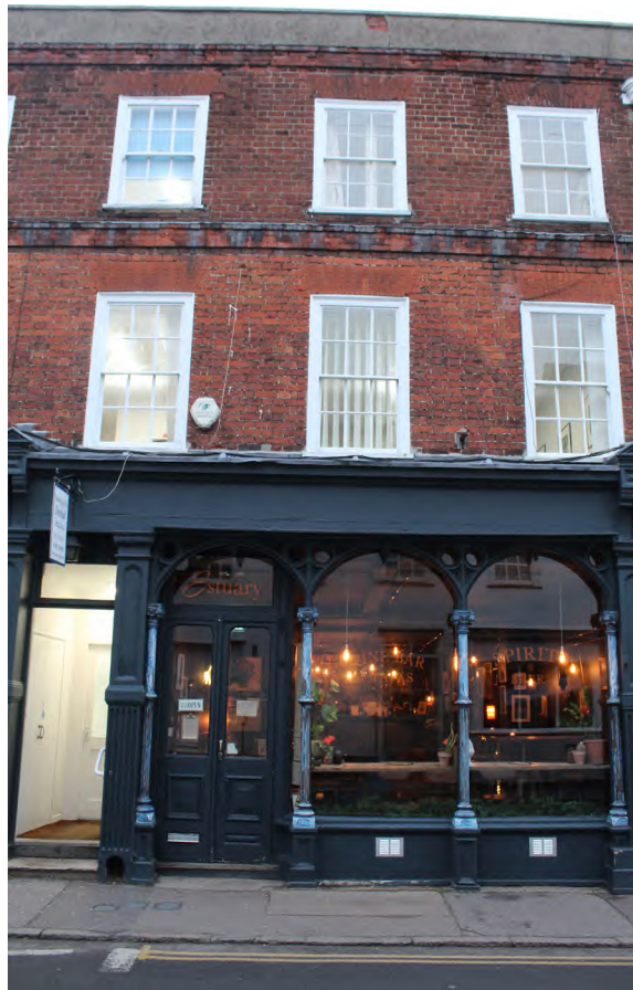
Figure 147 Historic shop frontage, Manningtree
