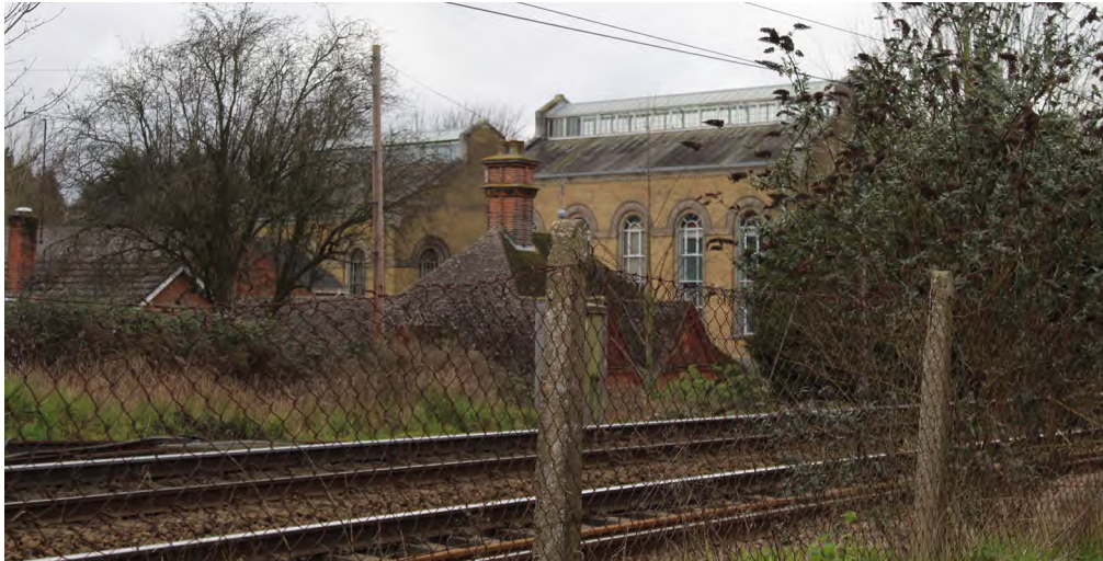
Figure 69 Pump House and railway, Lawford Water Works
