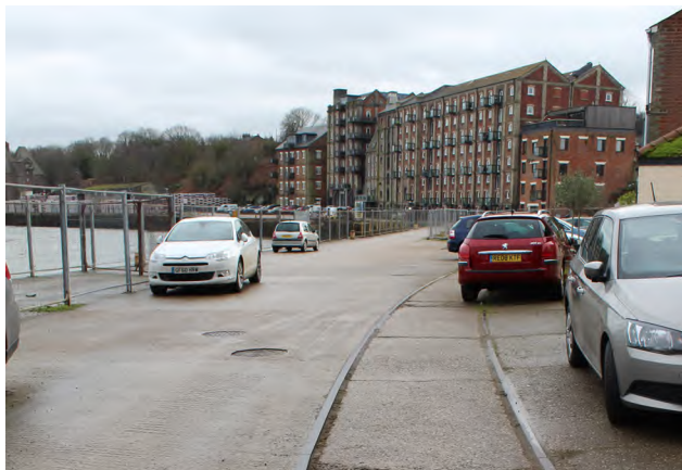
Figure 110 Surviving rails of the tramway which once spanned the quayside at Mistley
