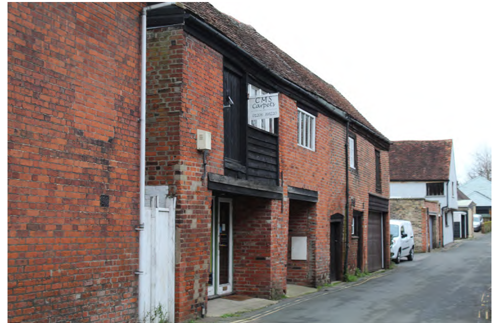
Figure 49 Industrial buildings on Stour Street featuring repaired brickwork and black weatherboard infill
