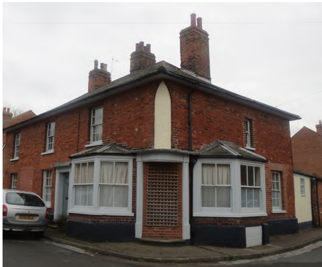
Figure 126 Former Lord Denman Inn, California Road
