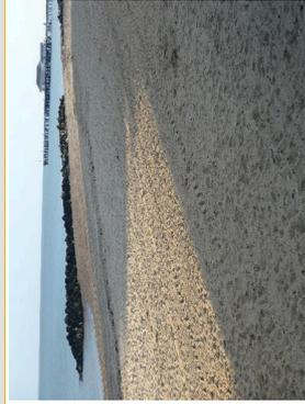
Noticeably there is more sediment around the end of the rock groyne to the north than the one in the south. This suggest the coastline has experienced longshore drift in a northwards direction here.
