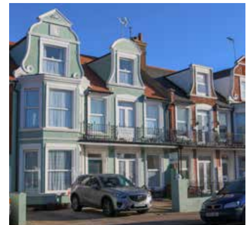
Figure 42 Agate Road (looking East)
