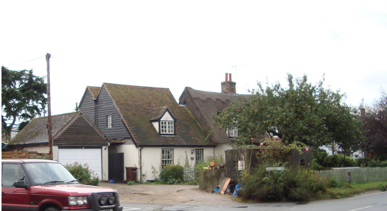
Figure 24 Apple Tree Cottage and No. 2, High Street with pillbox in foreground
