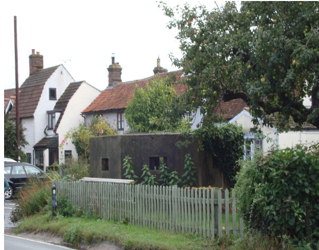
Figure 17 Pillbox outside Apple Tree Cottage, High Street
