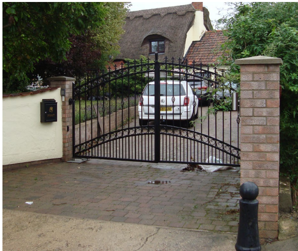
Figure 48 Inappropriate modern metal gates to a vernacular dwelling on Farm Road
