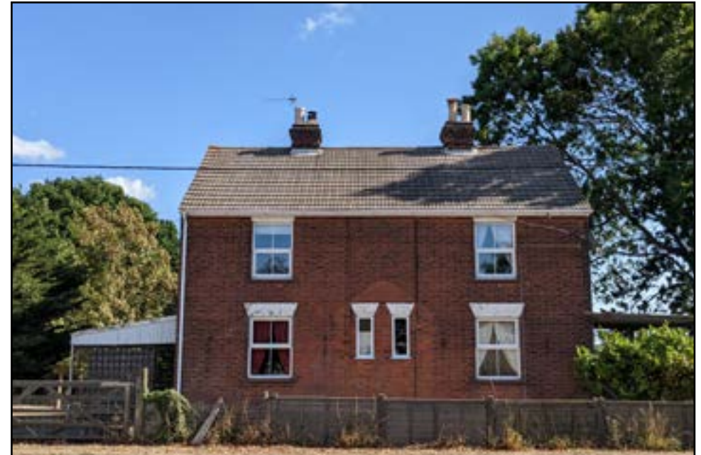
Figure 2 Buildings on Church Road
