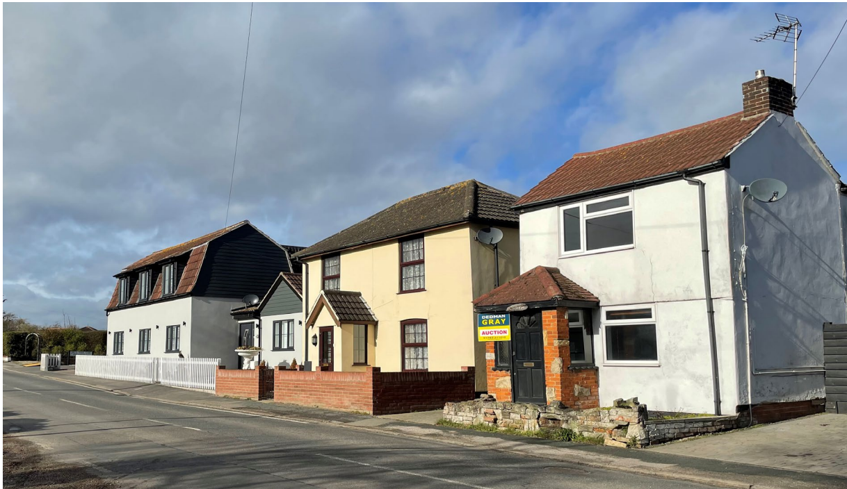
Figure 29 Row of residential cottages Numbers 64--60 located opposite Mumfords Lane
