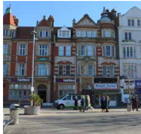
Figure 25 Natwest Bank Building
