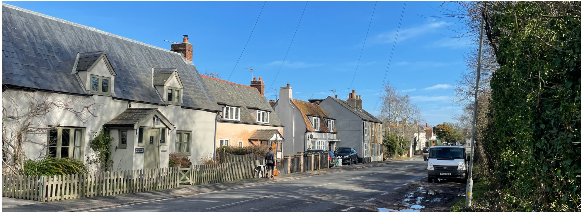
Figure 47 Photograph from The Street towards the centre of the conservation area
