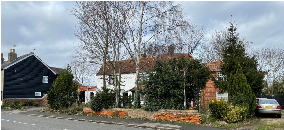
Figure 16 Photograph of Grade II listed Red House White House
