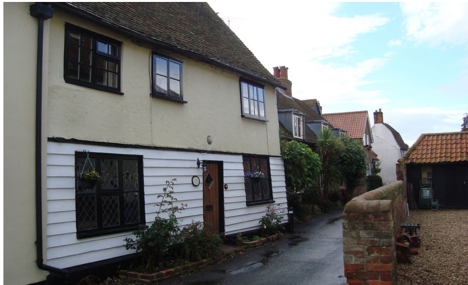
Figure 28 Vernacular materials including painted render, weatherboarding, clay tiles and pantiles and red brick boundary walls
