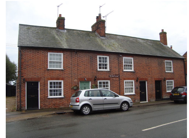
Figure 18 Mill House Cottages (2-5 High Street)
