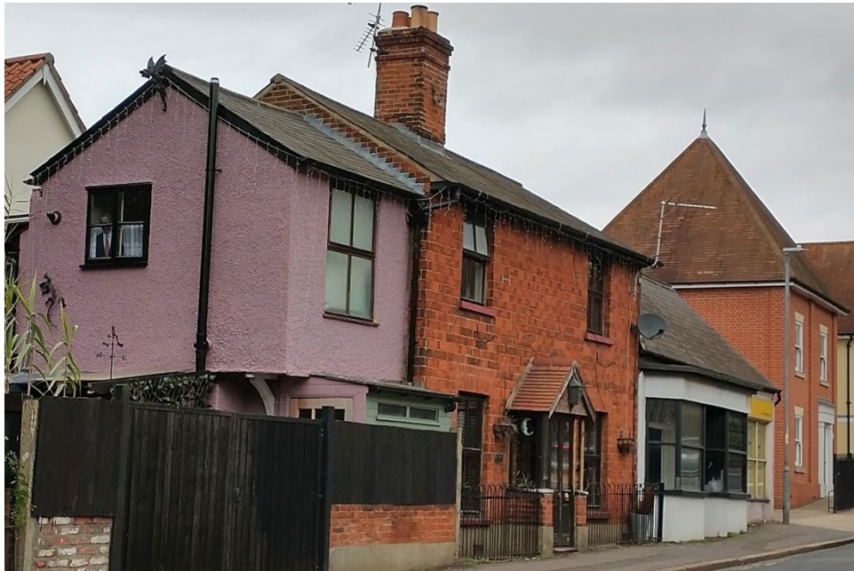
Figure 24 Number 395 Old Road in red brick laid in Rat Trap bond, with numbers 399 and 397 to the north
