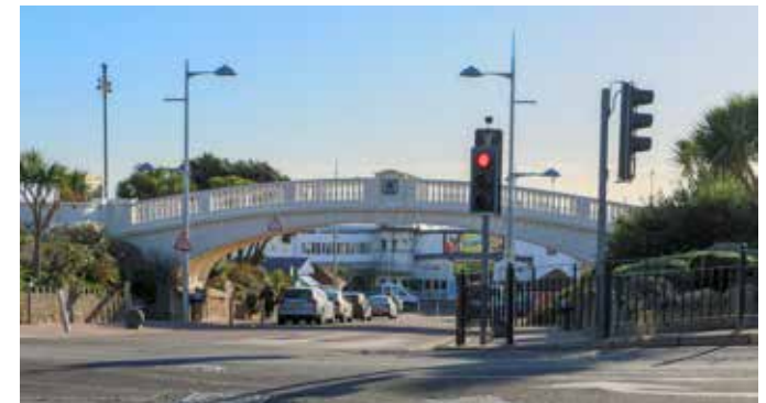
Figure 21 Pier Gap Bridge (looking South)
