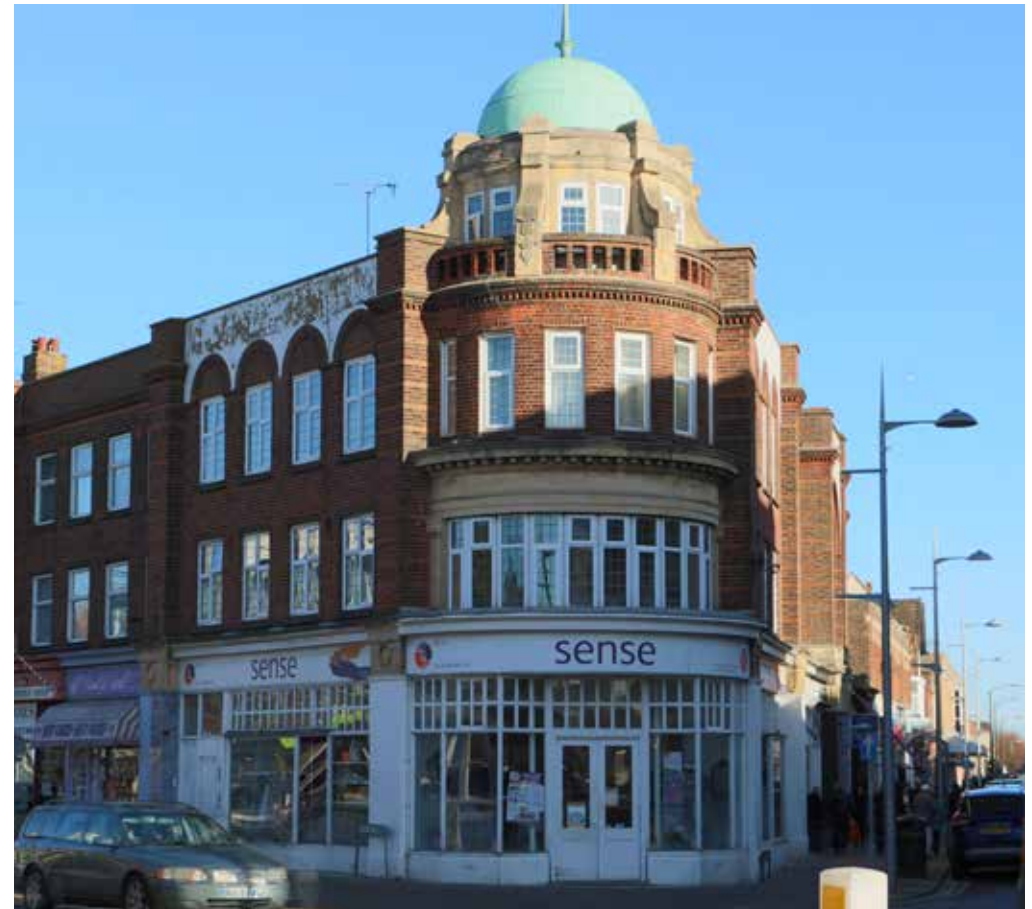
Figure 28 Corner building of Station Road and High Street
