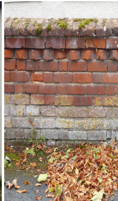
Figure 33 Traditional low brick wall surrounding the church hall
