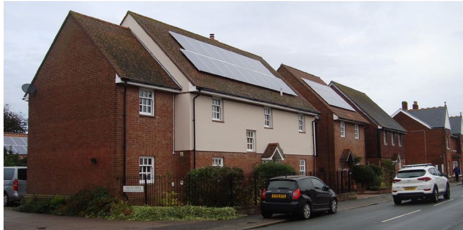
Figure 54 Modern development on the north side of the High Street
