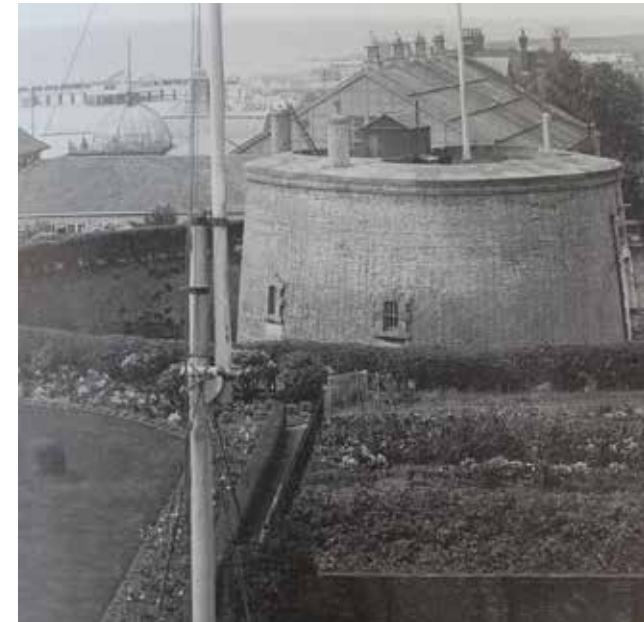
Figure 13 The Martello Tower (Britain in Old Photographs 1995)
