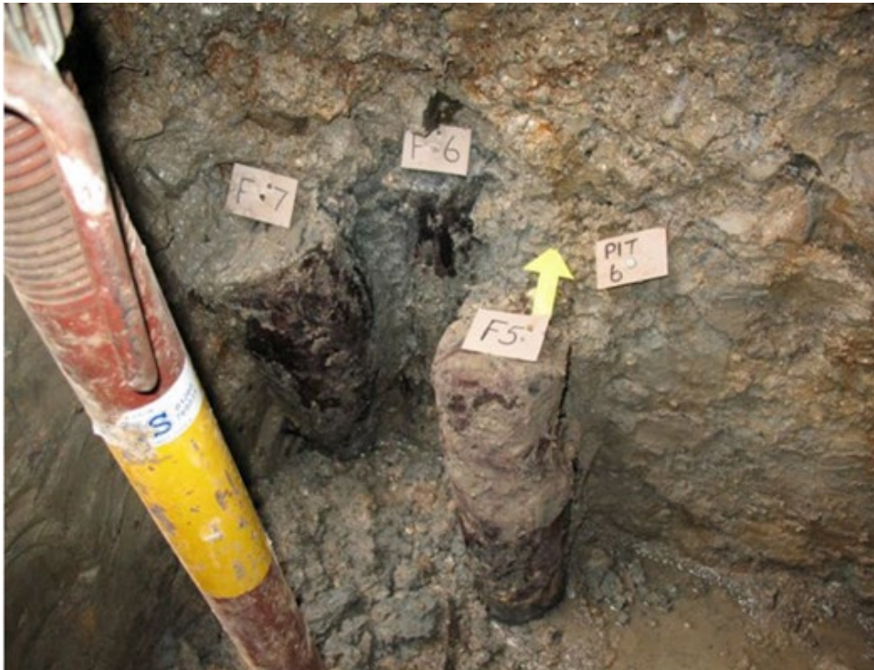
Figure 3 Three wooden piles beneath church tower.
