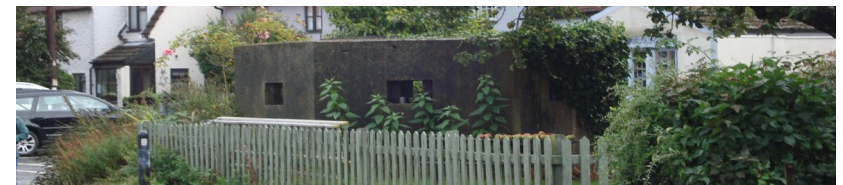
Figure 35 Pillbox outside Apple Tree Cottage, High Street
