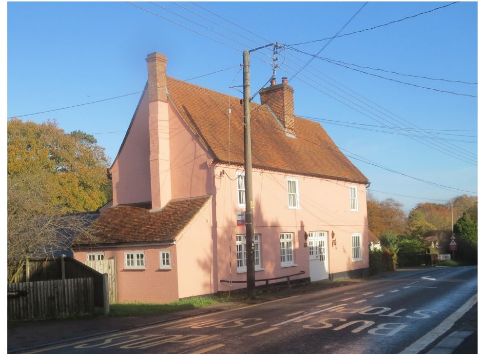
Figure 14 Photo of Kings Arms
