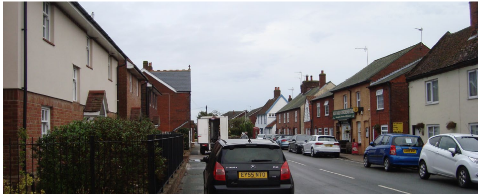
Figure 52 Car parking along High Street blocks the pavement in some areas
