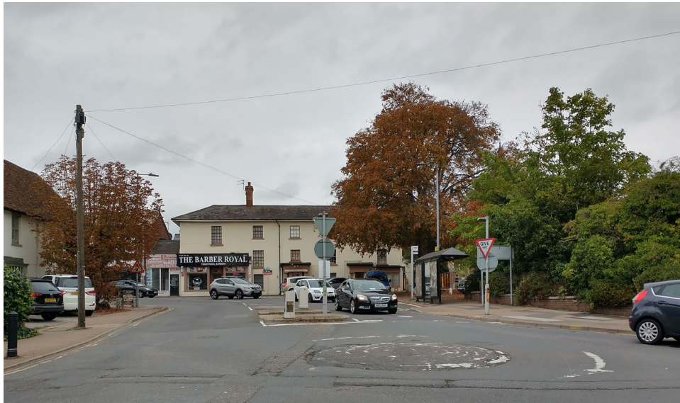
Figure 32 Poor quality surfaces and street furniture detract from the character and appearance of the Conservation Area
