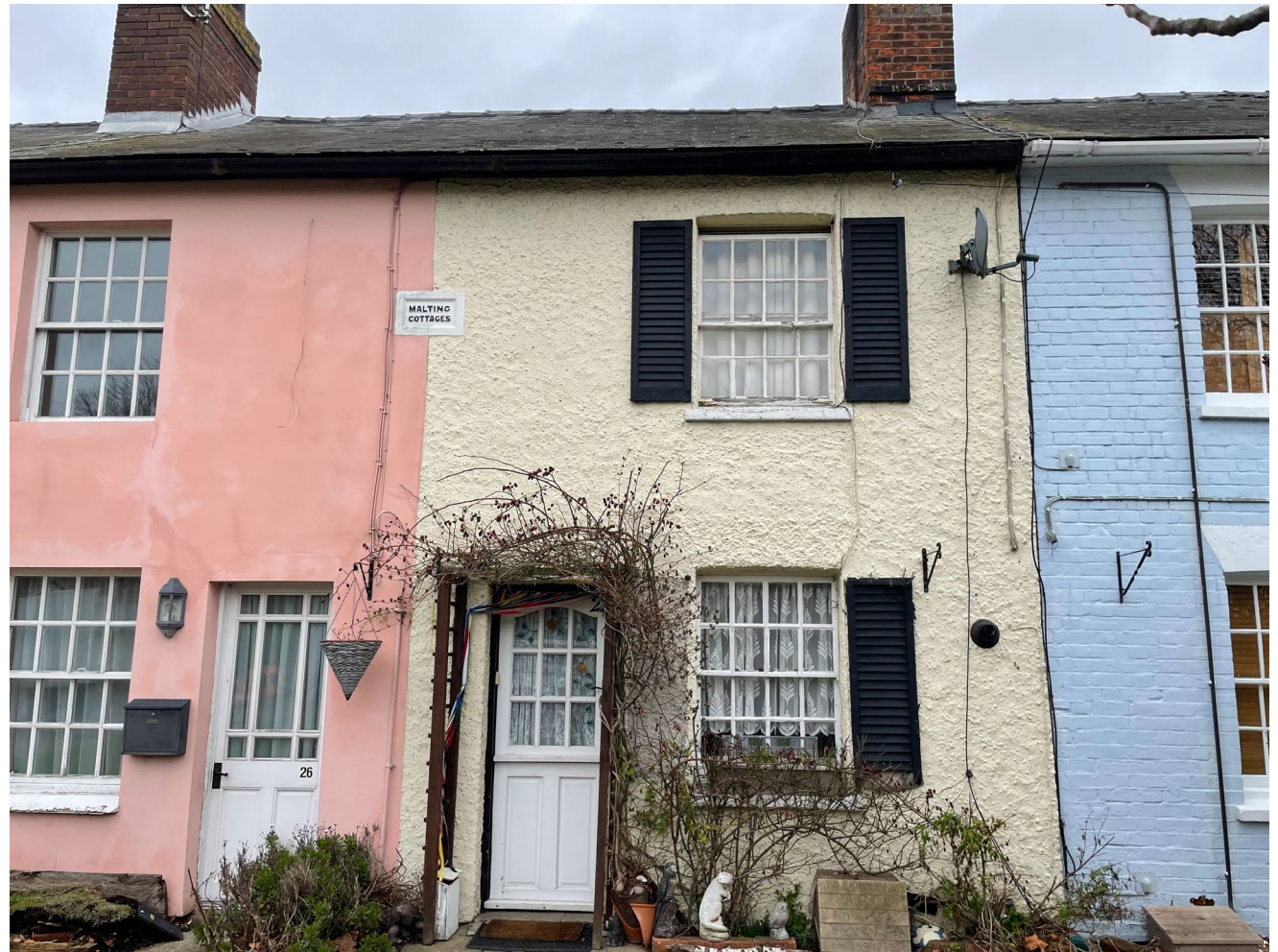
Figure 21 Close up of maltings Cottages
