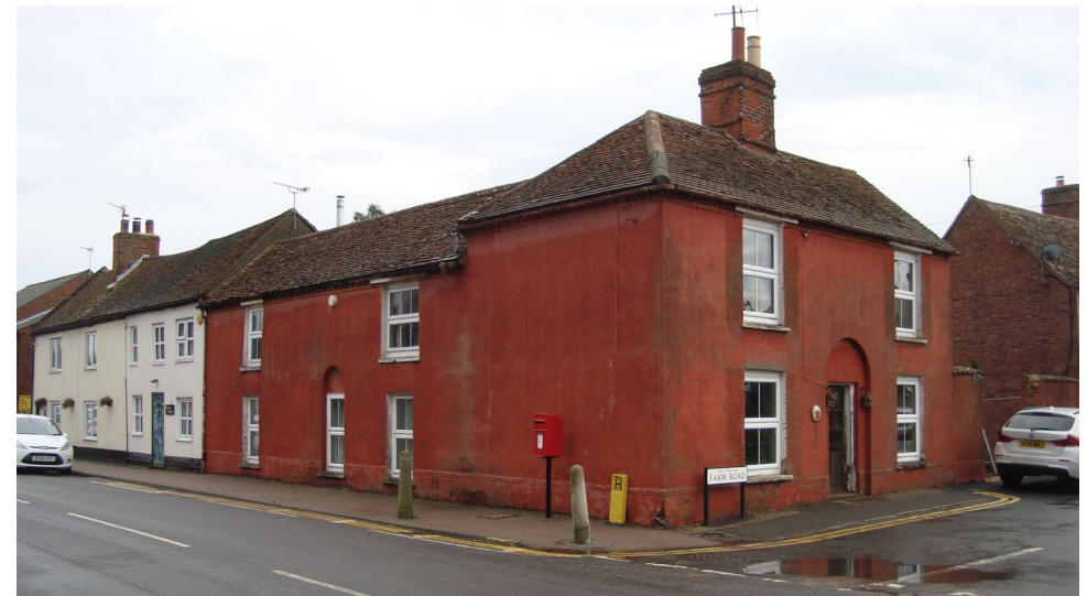
Figure 46 The insertion of inappropriate uPVC windows has harmed the historic and architectural interest of the Conservation Area
