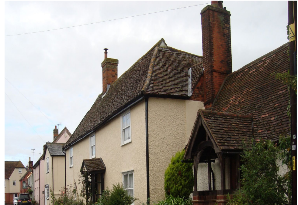
Figure 31 Grade II listed Maltings Farmhouse, a timber-framed and roughcast rendered house with fifteenth-century origins
