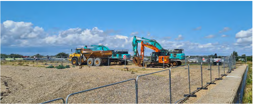
Fig. C13. Photographs of current works at Cockett Wick showing extent of plant and storage required for wall raising and defence reinforcement works.
