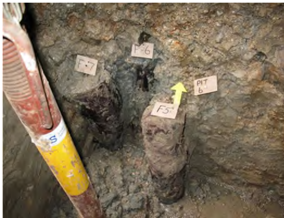
Figure 3 Three wooden piles beneath church tower.
