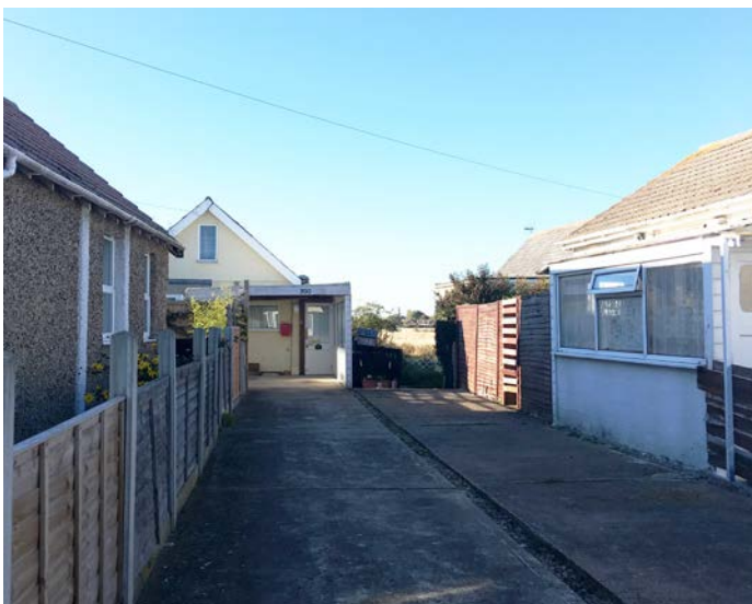
Fig. 43. Example of the relationship between the front and rear houses on the tandem plots
