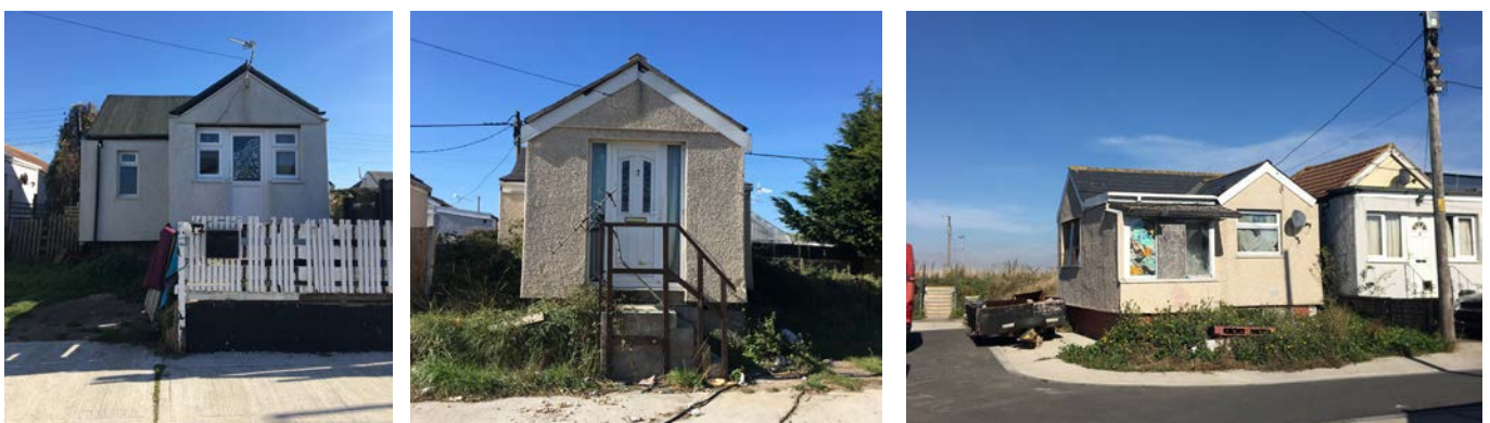
Fig. 48. The original chalet forms can still be found but in these examples, the overcladding in pebbledash has removed much of their charm and detail.
