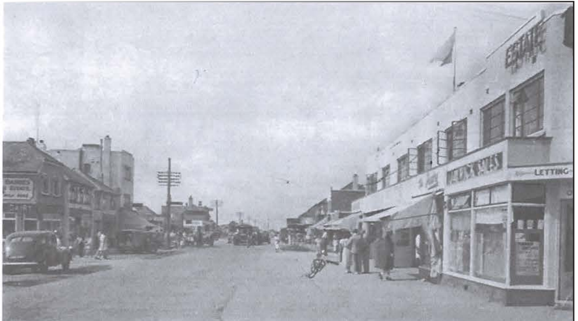
Fig. 40. Historic photo of Broadway - the building on the right is now Wonderland
