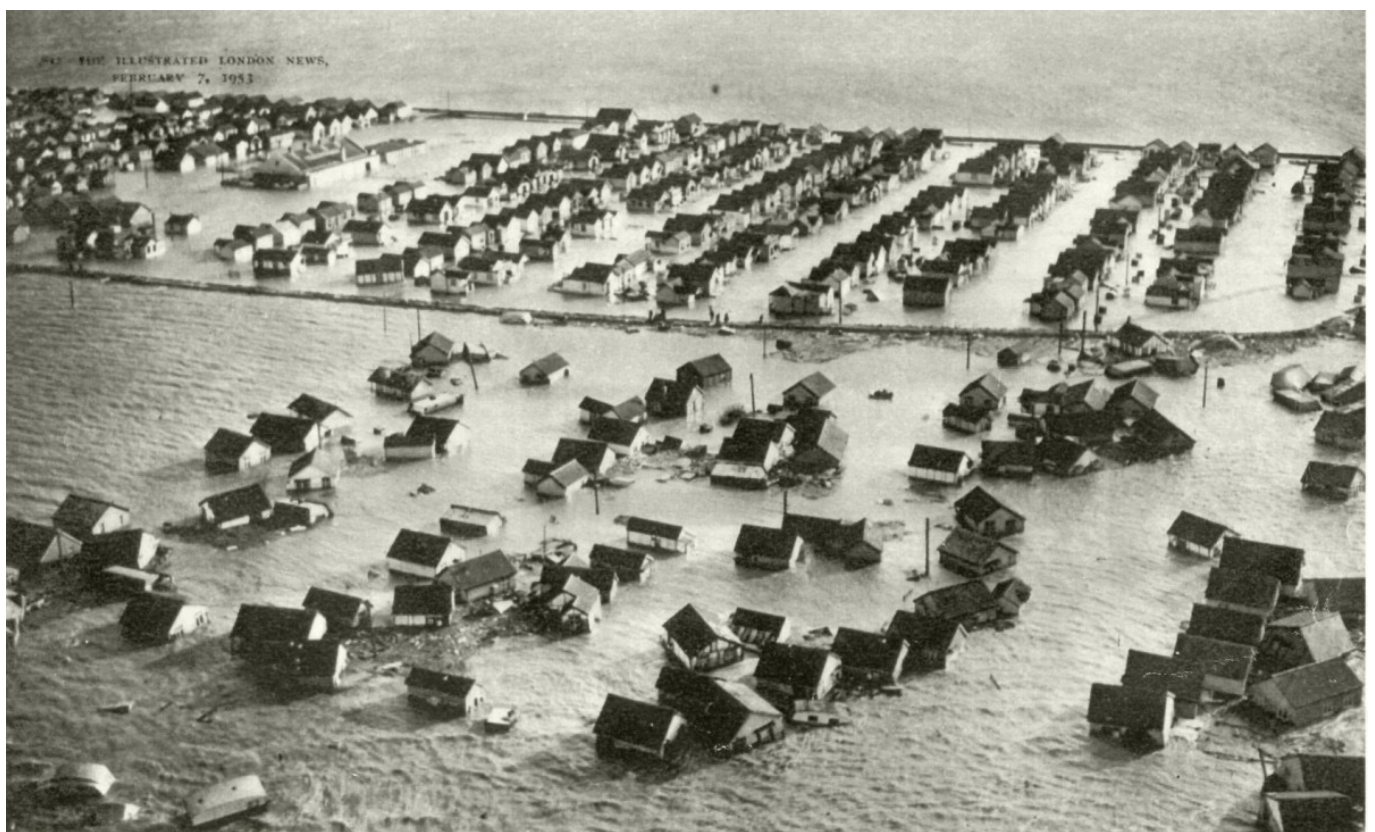
THE ESSEX BUNGALOW TOWN OF JAYWICK, NEAR CLACTON, AFTER THE SEA HAD SWEEPED OVER IT : 600 PEOPLE HAD TO TAKE REFUGE ON ROOFS AND SUN BALCONIES UNTIL THEY WERE RESCUED BY SMALL BOATS, AFTER THE FLOOD-WATER HAD SWIRLED INTO THEIR HOUSES ; AND THIRTY-FOUR WERE ON FEB. 2 REPORTED DEAD.
