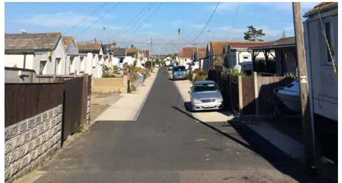
Fig. 14. Typical junction between Brooklands and north-south streets.
