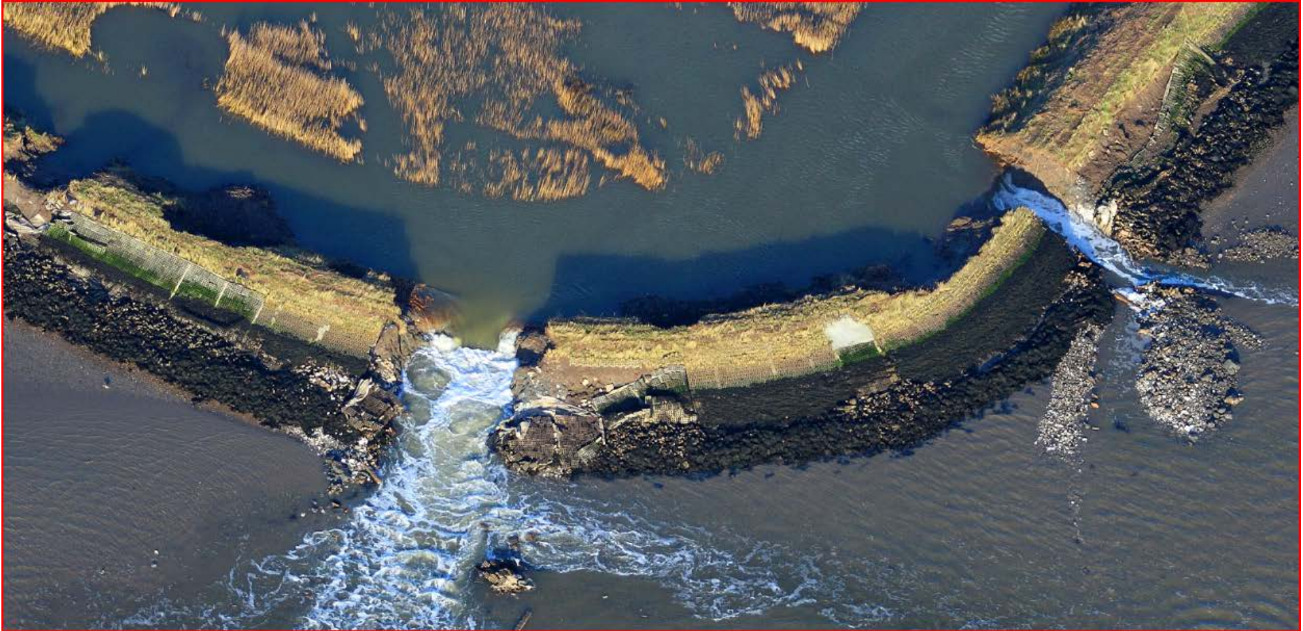
Photo 5 - Water ebbing out of marsh following a breach in sea defence near Aldeburgh, Suffolk – North Sea Tidal Surge Dec 2013 (photo provided by the Environment Agency)
