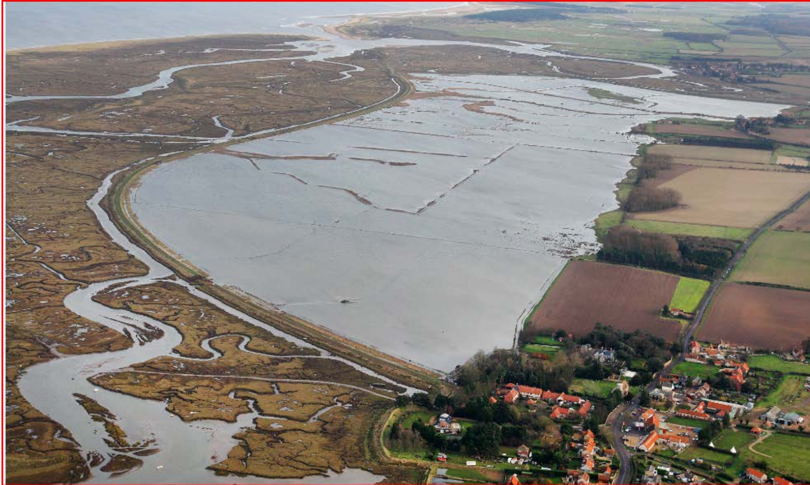
Photo 6 - Extent of land flooded following embankment breach, Burnham Deepdale, Norfolk – North Sea Tidal Surge – Dec 2013 Note: This area is topographically very similar in nature to St. Osyth Marsh (Hutleys, Bel-air, Martello, Seawick, St Osyth Beach) – (photo provided by the Environment Agency)
