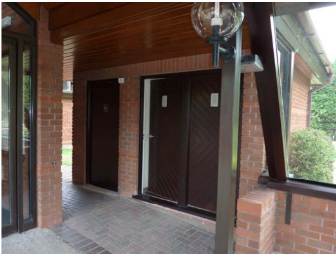
Showing existing public WC facilities (next to the flower tribute area)
